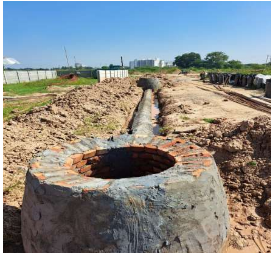
Sewer Line (Manhole Construction)
